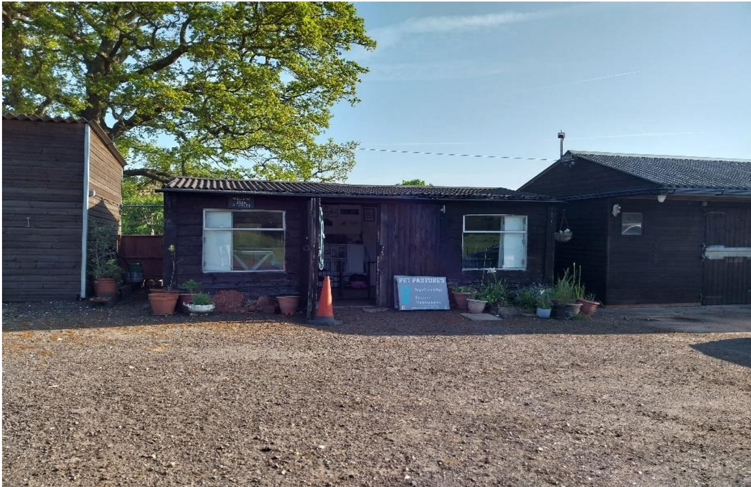
Photo - Front elevation of building
